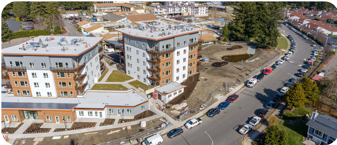
The two Villas on the left, with the Service Center and new Apartment building in the background, as seen from Highlands Parkway. Photo taken March 2023, courtesy of Walsh Construction Co.
